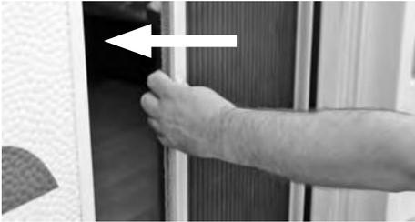
Always hold the rail in the middle to operate the insect screen door and pull it across the entire width of the door opening.
