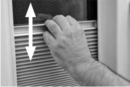
Always hold the pleated shade's top rail in the middle and move the shade up or down until you have achieved the desired degree of shade. Avoid slanting or tilting the rail when pulling it.
